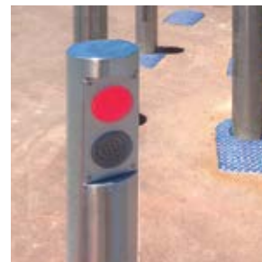
Above, use of traffic light bollards at a busy access point and left, exterior cabinet with compressor and logical controller.
